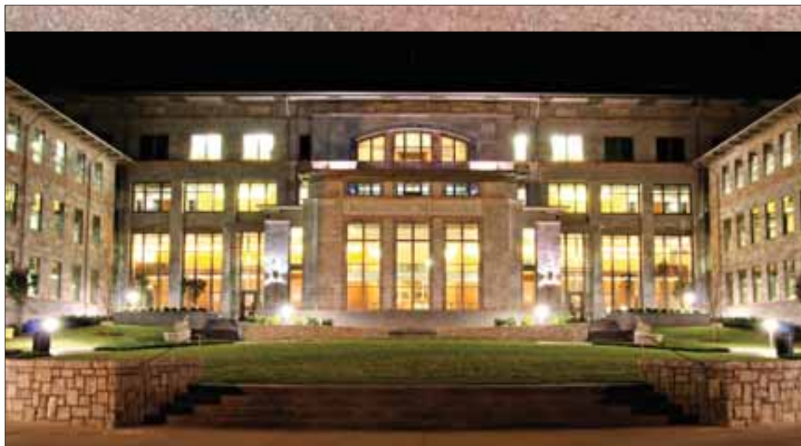
25,000 square feet of Polycor White Cherokee, Pearl Grey and Etowah Fleuri marble was used for the exterior of the Emory School of Medicine. In addition, over 12,000 square feet of Polycor White Georgia Marble was for the other two wings pictured above.
