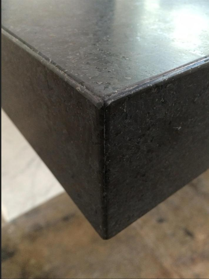
The counter appears as a solid block of stone but is actually 1 cm Ultra-Thin slabs of Cambrian Black **honed** granite, mitered over a plywood substrate
