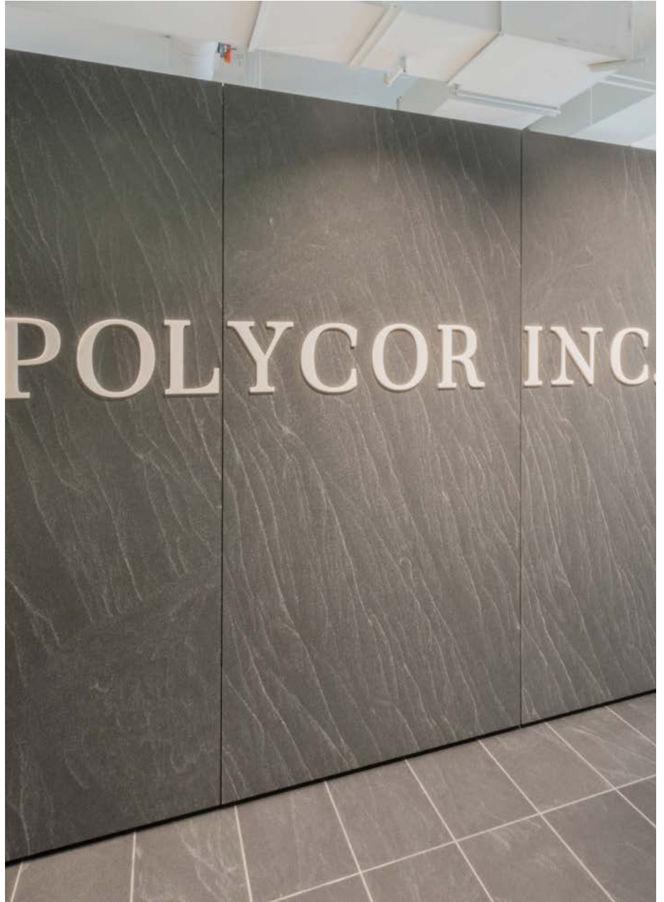
AMERICAN BLACK® granite, Eclad system installation, antique finish AMERICAN BLACK® granite, tiles, antique finish
