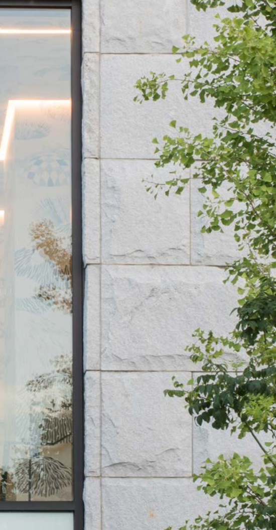
Vertical application, rock pitched finish
