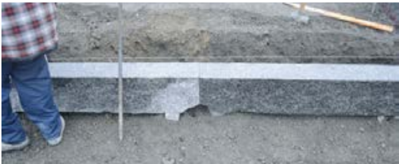
The sawn ends allow for easy jointing of the curbs, eliminating the need for mortar grouting.
