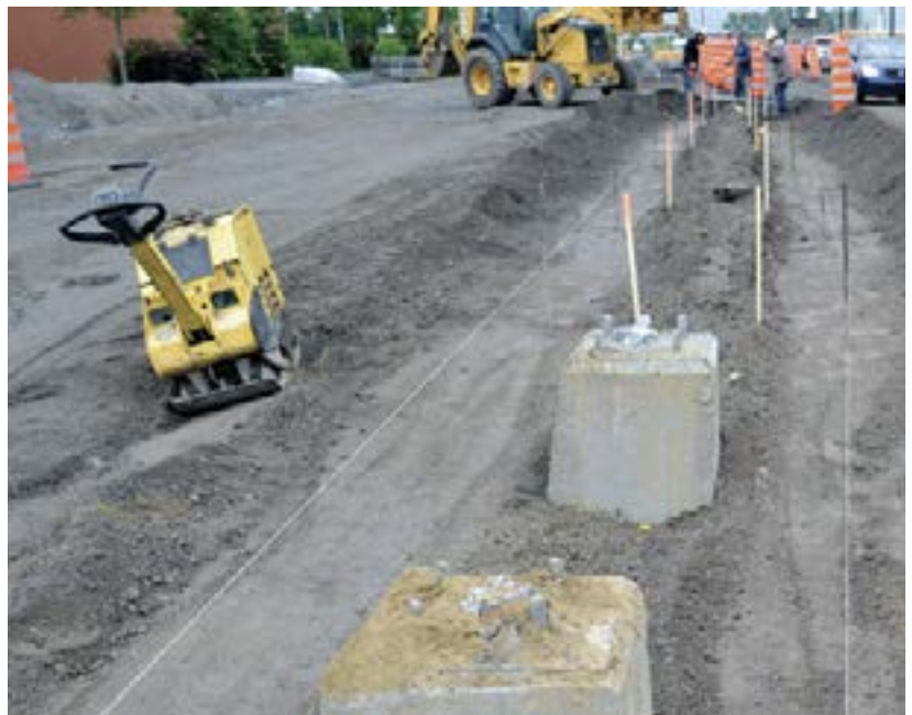
The crushed stone base course is mechanically compacted to a density of 95%.
