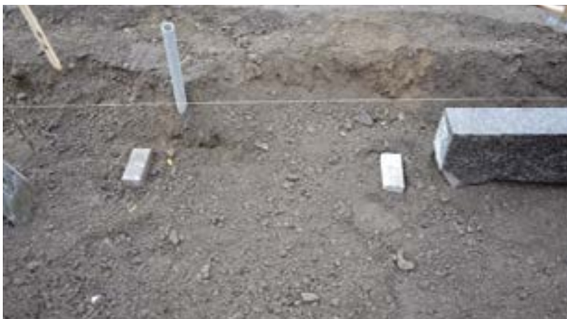
Concrete wedges on which the granite curb will rest.
