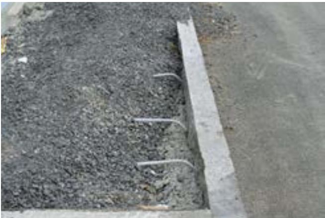
Curbs with anchoring system to sidewalk.
